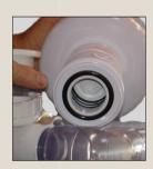
Install a #8 standard rubber winter plug in the opening where the Vac- Alert<sup>™</sup> SVRS was located.
